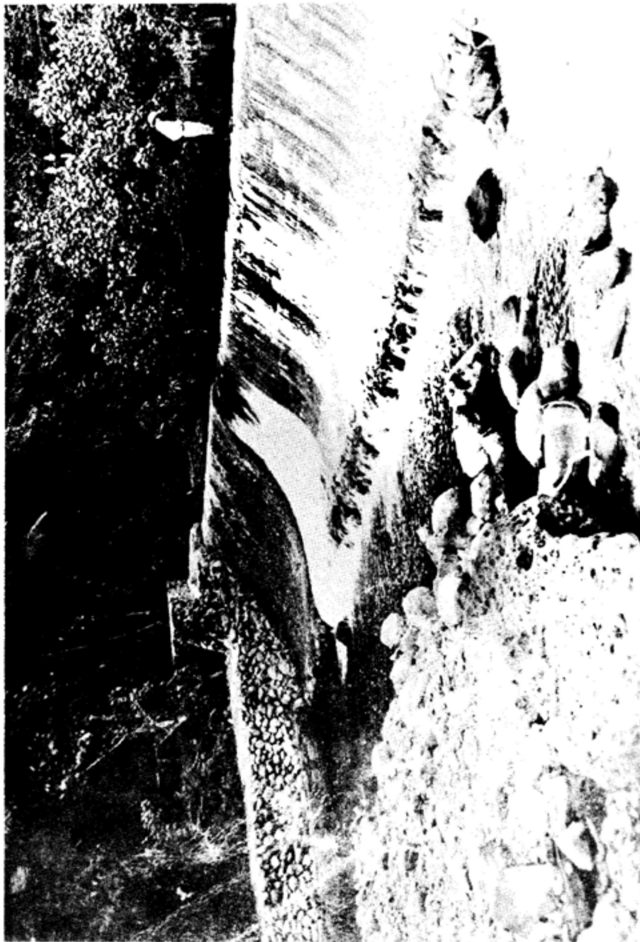
A Japanese built dam in Ponape: the dam was part of a scheme to use Ponape's rivers and waterfalls as parts of a water-powered electrical plant.
